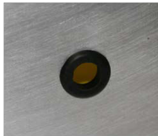
Wall Penetration with Grommet Installed
